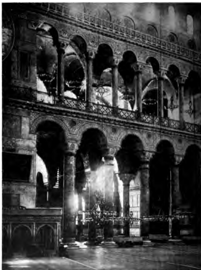
GROUND STORY AND GALLERY ARCADES FROM NAVE Santa Sophia, Constantinople
